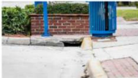
Image 11 – Bulb out drain are clear and free of debris.
